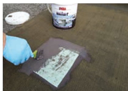
RESTORATION OF ANCIENT BITUMINOUS MEMBRANES
